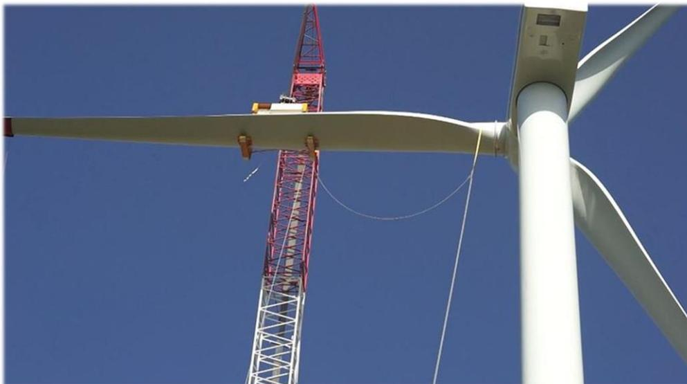
Figure 3: Wind turbine generator assembly
